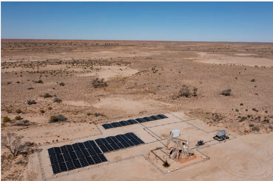
Gas mining rig in the south Australian desert powered by solar energy. Source: iStock
