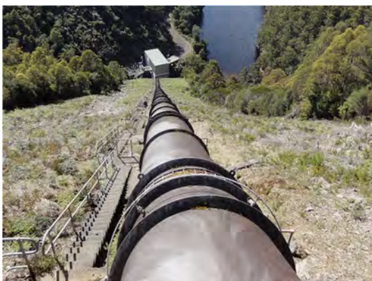
Two hydro-electric plants in Tasmania. Left. Wilmot power station, 32 MW. Water flows down the pipe to the turbine in the building at the bottom. Right: The Gordon Dam, 450 MW. Three underground turbines are fed from an 80 m vertical channel from the bottom of the lake.
