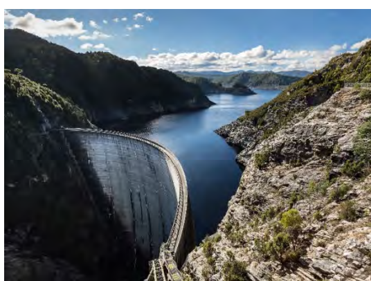
Two hydro-electric plants in Tasmania. Left. Wilmot power station, 32 MW. Water flows down the pipe to the turbine in the building at the bottom. Right: The Gordon Dam, 450 MW. Three underground turbines are fed from an 80 m vertical channel from the bottom of the lake.
