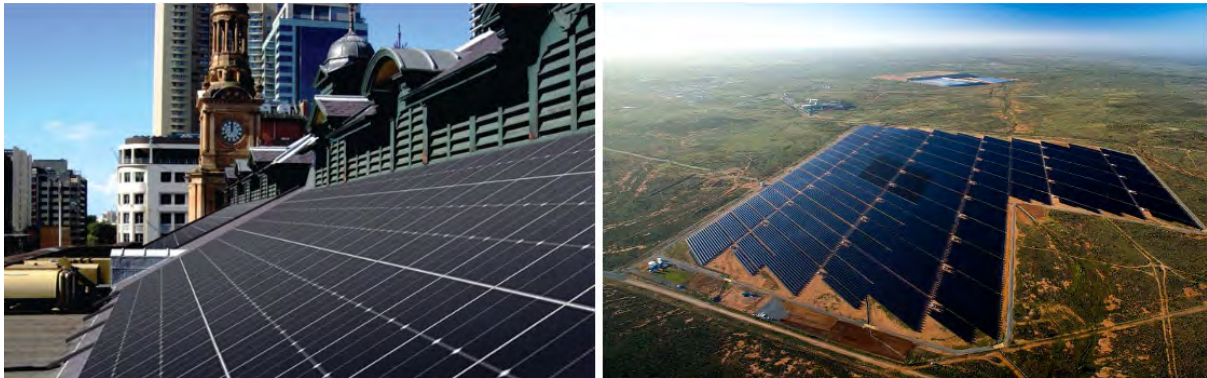
Solar panels on the Sydney Town Hall, and the 53 MW Broken Hill Solar Farm, which covers 140 hectares.
