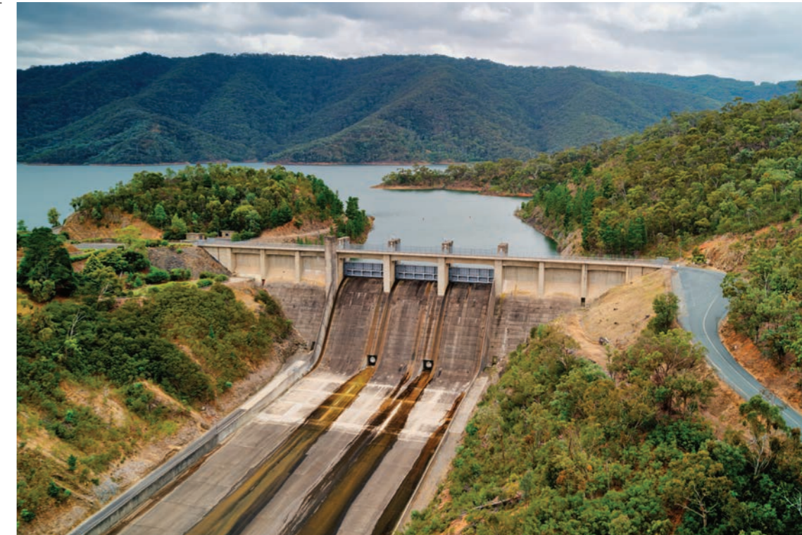
RIGHT: Eildon Dam is a rock and earth-fill embankment dam with a controlled spillway, located on the Goulburn River between the regional towns of Mansfield and Eildon within Lake Eildon National Park, in the Alpine region of Victoria.
