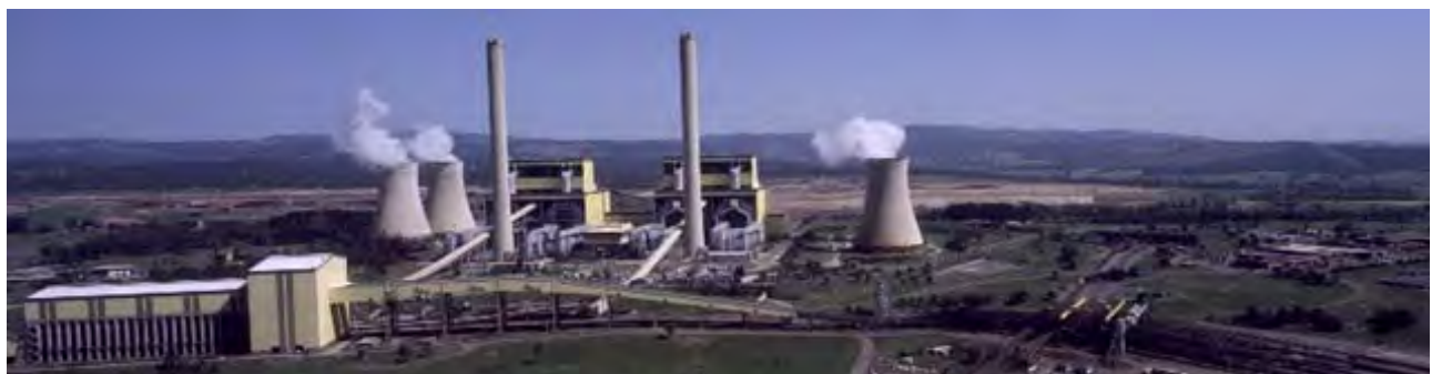
Figure 2 Another view of the Loy Yang coal-fired power station shown on page 73. The tall chimney stacks are above the furnaces. The huge curved towers with steam pouring from them, often mistaken for the pollution from the furnaces, are the cooling towers.
